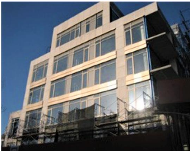
NYS BCP Project Ave. U Brooklyn Photo: Hydrotech
